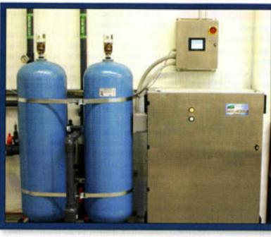
PROTECTION: The Eco-Safe **Dual MD-2000** is being used at Culver City Meat Co., Vernon, as a primary disinfection system. It incorporates dual ozone generating systems designed for flexibility in ozone demand/supply and backup redundancy.
